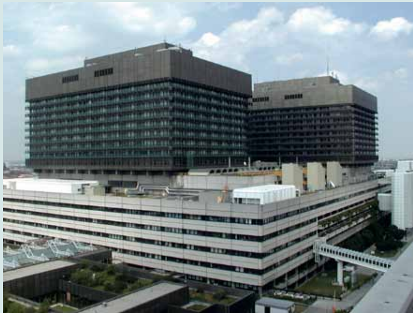
AKH Vienna (source: AKH information centre)
